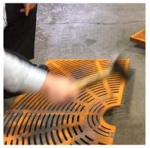
2. Repeatedly hit the grate at this spot with the mini sledgehammer.
