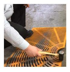
1. Remove the grate from the Filterra frame, place it flat on a hard surface, and support the grate by stepping on the edge or using other weighted items such as a few mulch bags if this is being done during a Filterra maintenance event. Put on safety glasses/goggles. Align the mini sledgehammer as shown in the figure to the left. The head of the sledgehammer should be aimed just inside the wide cast iron bar between the larger grate section and the breakaway section.
