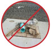
2. Final paving must be completed. Final paving ensures that paving materials will not enter and contaminate the Filterra system during the paving process, and that the plant will receive runoff from the drainage area, assisting with plant survival for the Filterra system.
