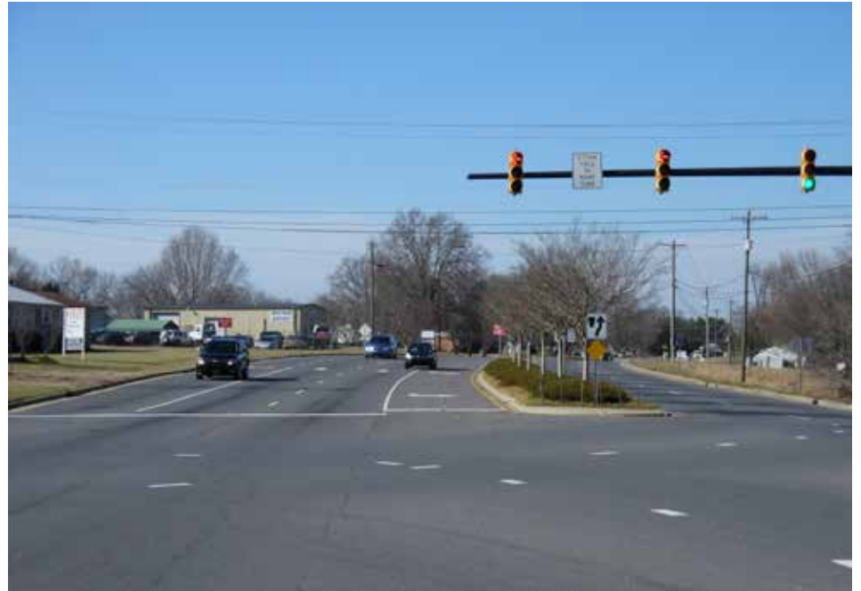
View of Kannapolis Parkway / Glen Afton Boulevard intersection looking north.
