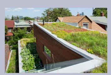
that can retain rainwater. They present an alternative to traditional roofs which typically contribute to the rate of runoff. In addition to controlling the quantity and quality of stormwater, green roofs provide other benefits, including building insulation (which results in a reduction in energy costs), heat island mitigation, and wildlife habitat. Green roofs may require extensive design considerations and maintenance.
