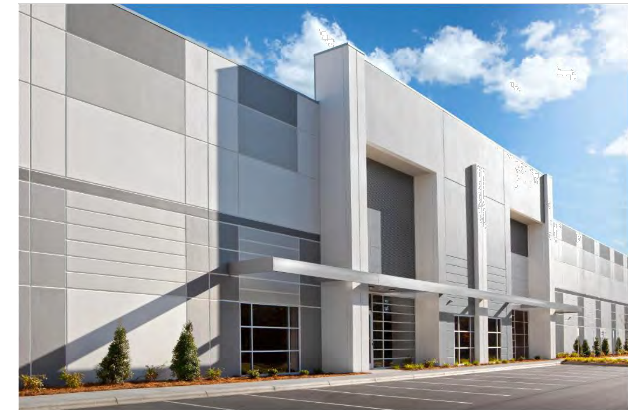
•Buildings shall have articulations in the overall massing that shall break down the building scale through use of offsets, recesses and varying materials
