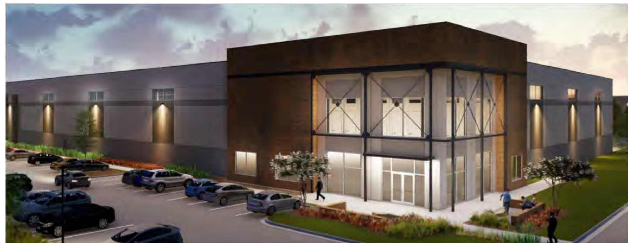
•Creation of visual layers with exposed steel, perforated metal or mesh screening / shading devices.
