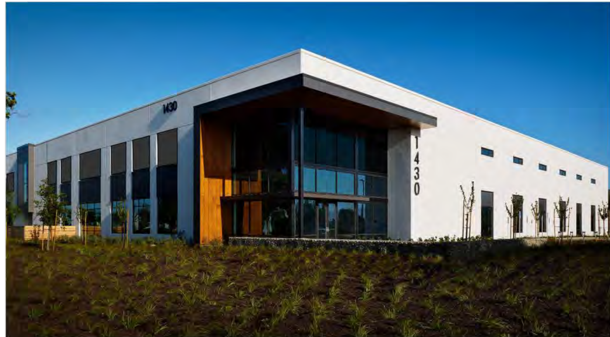
•Clear entry points will be highlighted through the use of offsets, canopies, overhangs, illumination and prominent detailing. Articulation using varying opening sizes, materials, patterns, recesses and projections
