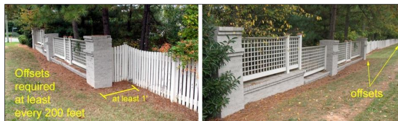
Figure 5.5.G: Fence and Wall Offsets
