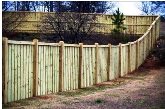
Figure 5.5.H: Fence with Finished Side Out
