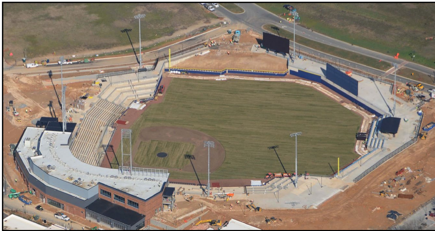
SEV Construction Progress: January 2020
